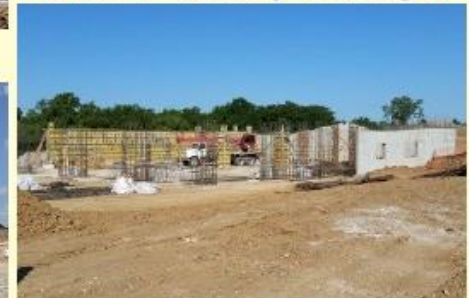
July 7 - Three Walls Up
