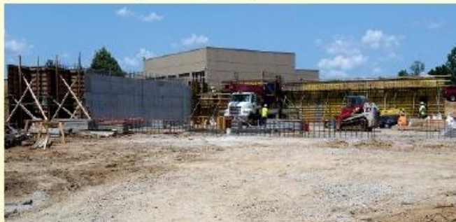
June 15 - Another Wall Up
