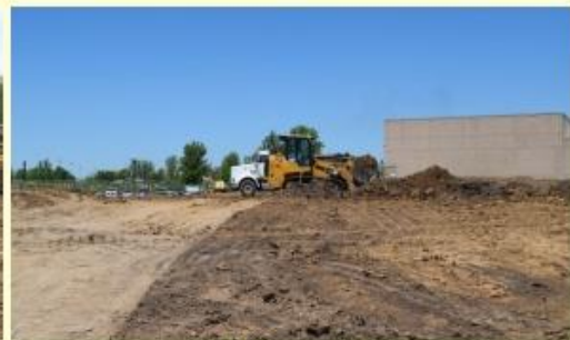
May 9 Leveling the Hill
