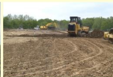
May 9 Grading Begins
