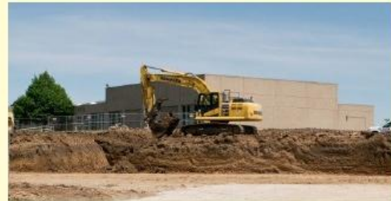
May 10 - Site Cleared
