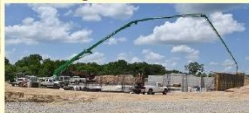
June 18 - Pouring Concrete
