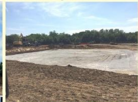
June 1 - Ready to Begin
