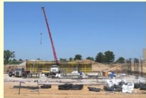
June 11 - First Wall Up
