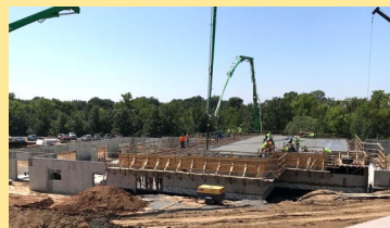
September 7 Pouring the Upper Level Slab
