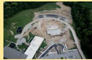
August 29 - Aerial View Construction Site
