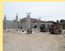
July 17 - Supports for Upper Level
