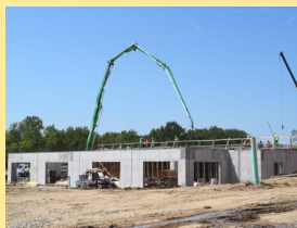
August 19 Pouring Concrete
