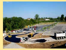
July 20 Construction Site
