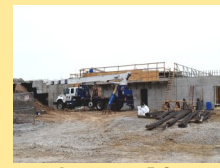
August 19 Forming Up Upper Level
