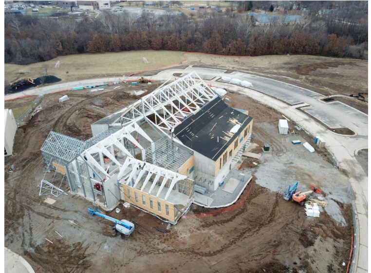
Multi roofs, all in various states of completion.
