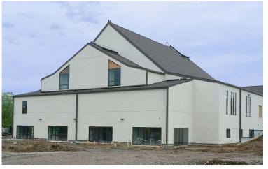
Despite difficulties with the mud we have finished the efis on the back (Eastern) portion of the church. The two upper windows, including the wood, will be replaced with stained glass. The ground will be graded north to south for runoff.
